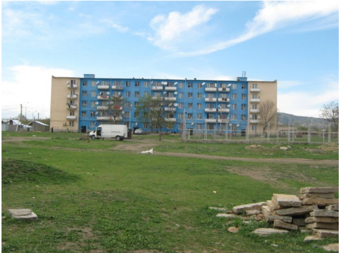
A building in Koda IDP settlement
