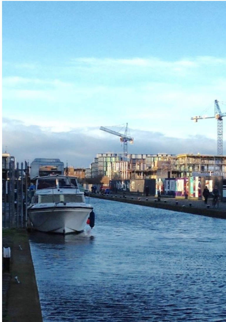
FIG 1: Construction on the canalside All photos © Authors
