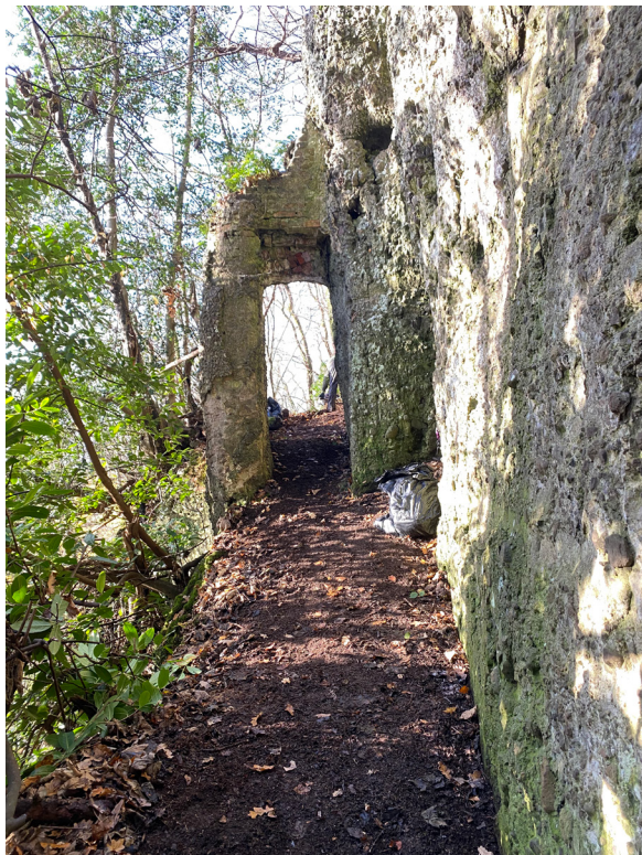
Figure 4: The doorway (Element A) from the east.
