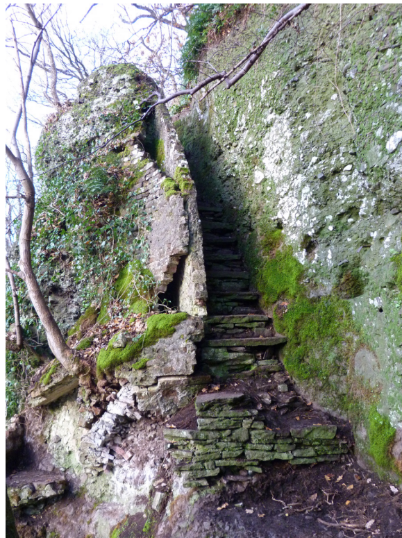
Figure 5: The staircase (Element C) from the east.
