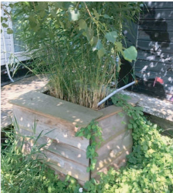
Figure 6: The bio-filters used to clean the water used in the houseboats (photograph by author)
