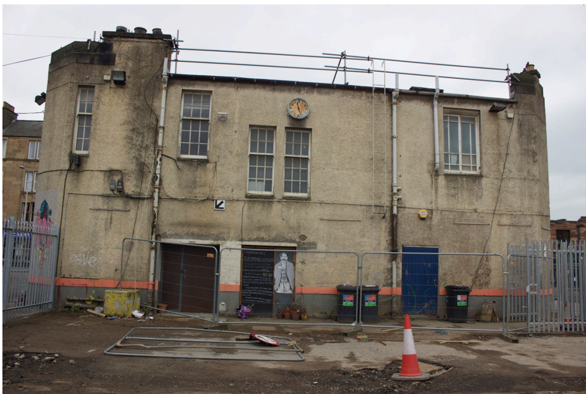
Figure 1. 165a Leith Walk from the back, where the trams were once housed. The figure of Ebenezer MaCrae can be seen on the middle rear doorway
