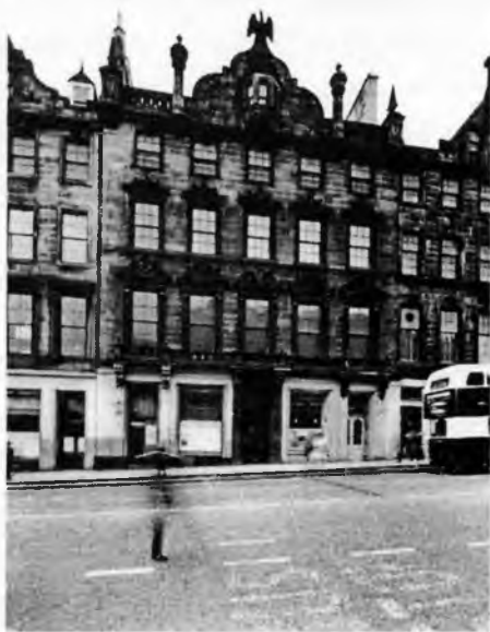
Figure 3. External view of the frontage of No. 7 Melbourne Place, showing the main entrance doorway, flanked on either side by two shops. The width of the Society's premises is seen to include the five windows clearly displayed on the 2 nd 3 rd and 4 th floors. The Eagle, with spread wings, is mounted on the pinnacle above the 5 th storey (with permission, Royal Commission on the Ancient Historical Monuments of Scotland).
