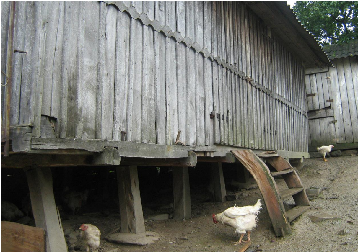
Figure 10. An example of a modern platform structure on sloped ground in the village of Răcățău.
