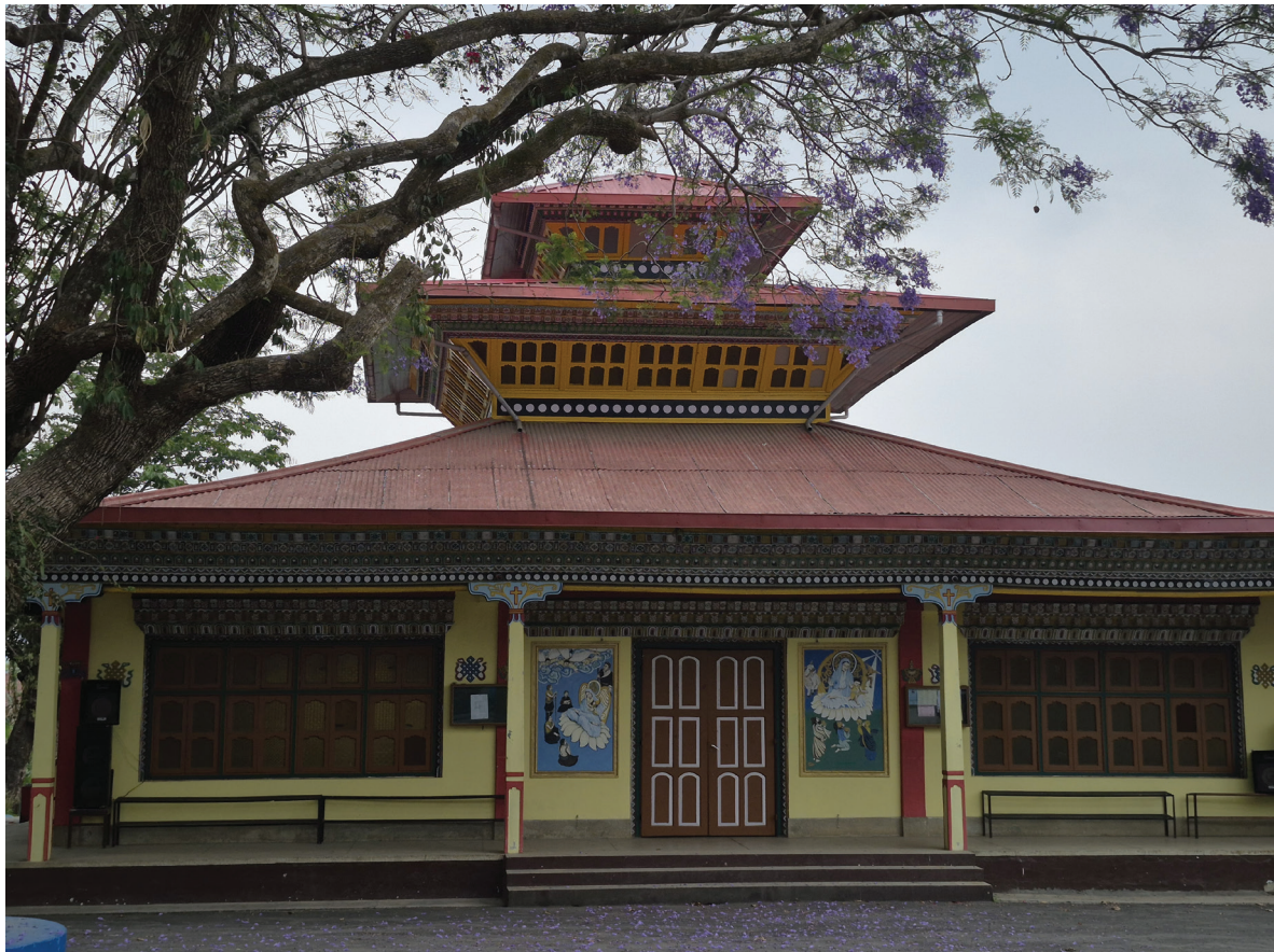
Figure 1. Mary Mother of God Church, Kalimpong, West Bengal. The multi-tiered roof and painted woodwork that lead many first-time visitors to take the building for a monastery. 24 April 2026. Photo: Tenzin Nyima Bhutia.
