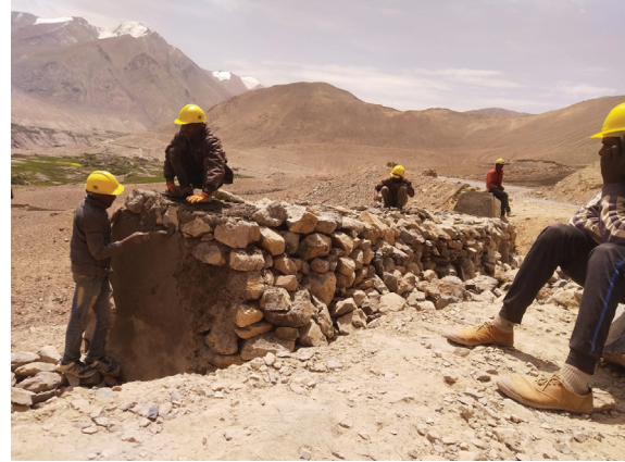
Figure 2. Building the Border Road. Road workers apply cement to a safety barrier while others rest, waiting for their turn. 2022. Photo: Prince Tomar.
