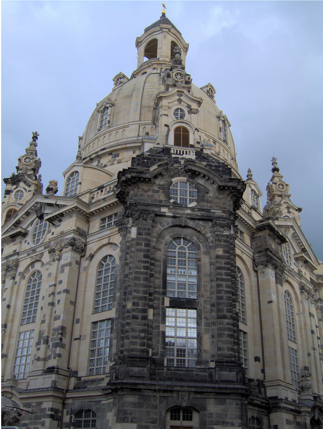
Figure 4: View of the Dresden Frauenkirche showing old (blackened) and new (light-colored) stone, 2006.
