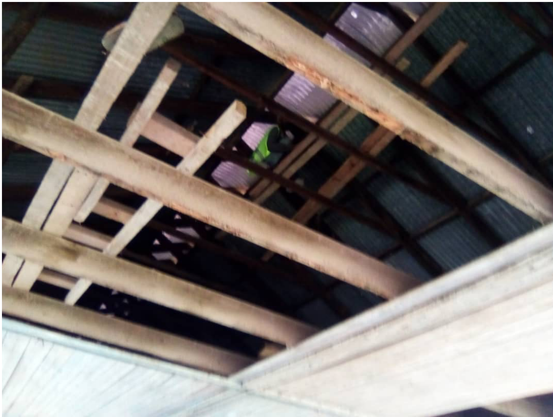
Figure 4: The artisans working on the felt underlay in the roof of the Premier Building. Photo taken by the author, 2023
