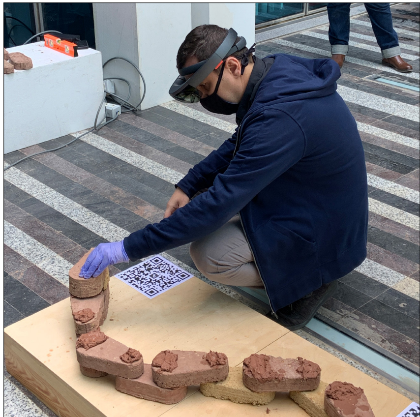
Figure 10. Bricklaying with earth mortar
