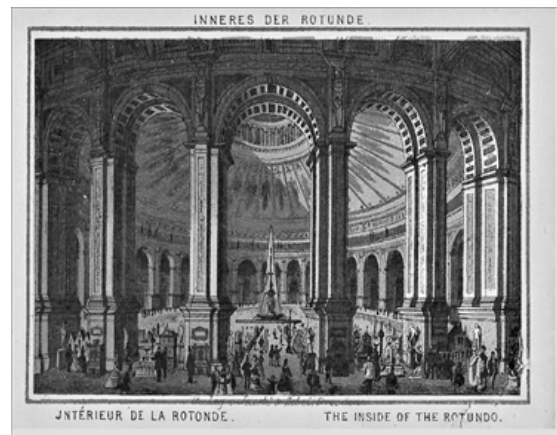
Figure 7. Interior of the Rotunda
